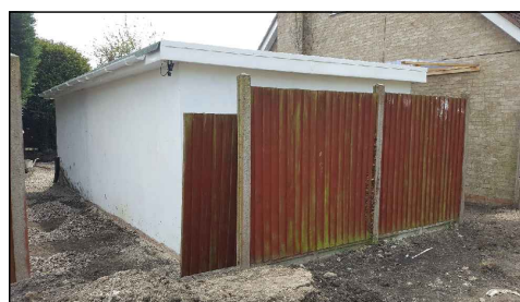
Photograph of outbuilding
