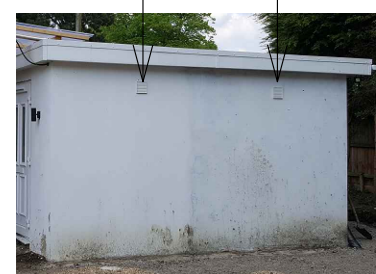
Photograph of south elevation of outbuilding showing extract positions
